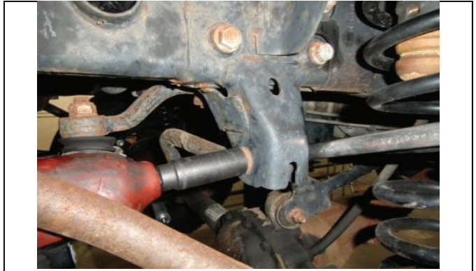
Support front axle and remove upper track bar bolt.
