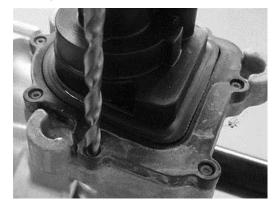
O Using a 1/8" drill bit, drill out all seven rivets.
