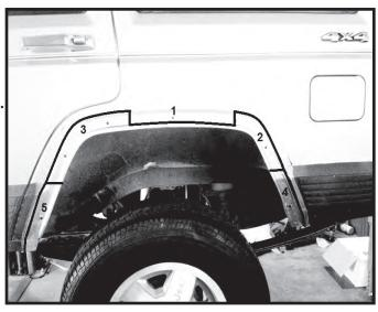
Step 35. Cut area # 4 carefully. Start by cutting 3/8 inch from the line and grind the rest of the way. A filler putty or silicone is needed to fill the gap between the sheet metal. Repeat for opposite side.
