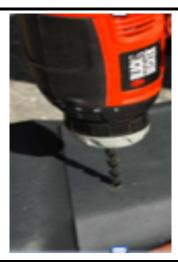
**4)** Using a 1/4" Drill Bit - Drill the installation holes using the Five (5) pre-drilled holes in the Bumper Cap as a guide
