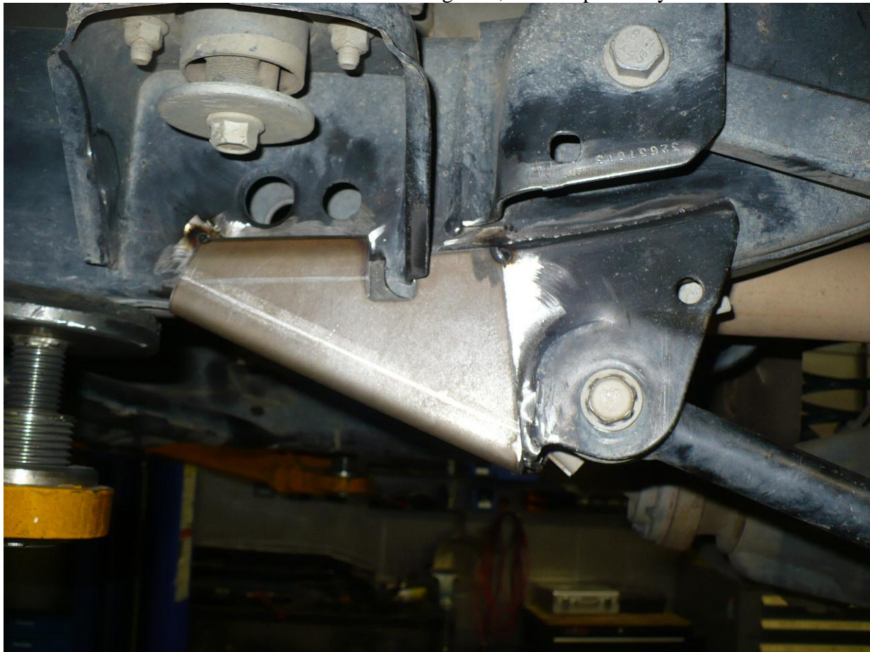
IMG. 2.2 Placement of 502202-01 RLCA outer gusset
