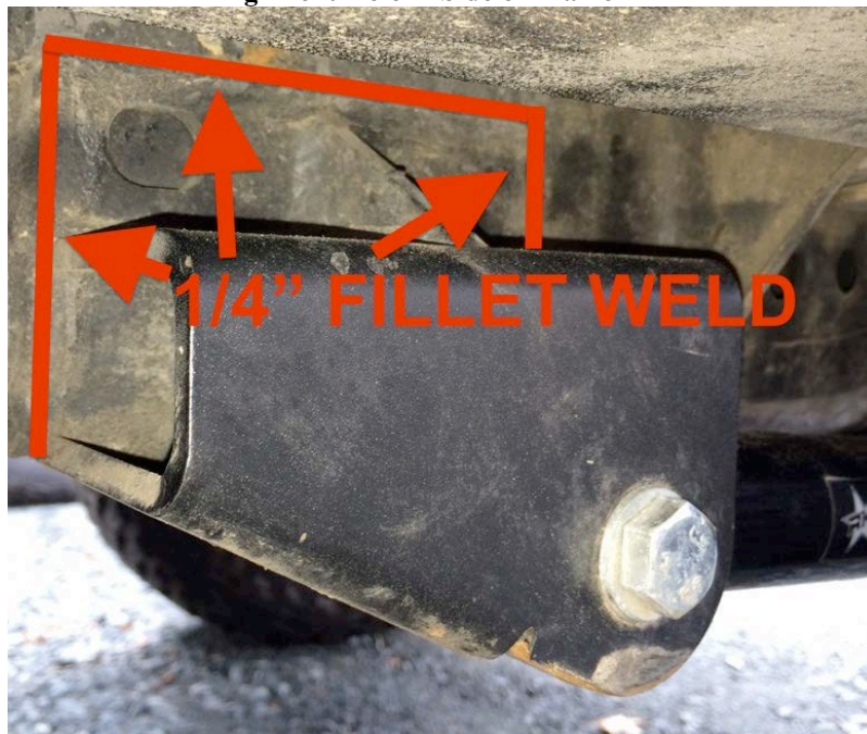
Weld on Lower Control Arm Mount
