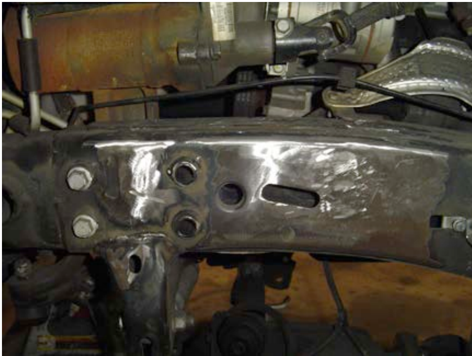
Driver's Side Frame Rail Showing Removal of OEM Spring and Shock Mount
