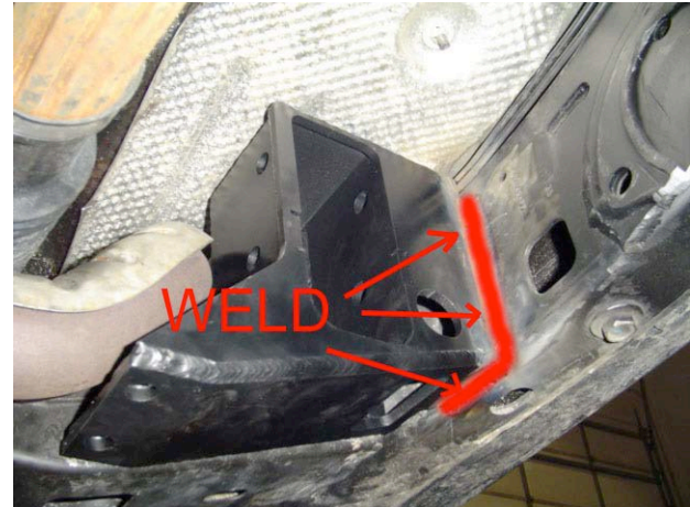
D.S. Bracket Welded in Place
