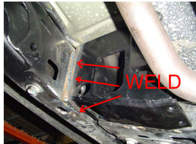
P.S. Bracket Welded in Place
