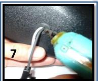
Gently pull excess wire from pods. We recommend sealing any airspace around wires with glue gun.
