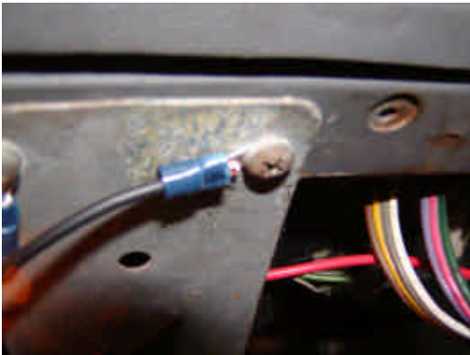
Figure 9. Terminals were crimped onto the Black ground wires and then they were placed under existing screws in the metal dash.
