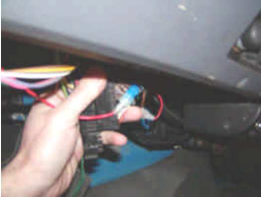
Figure 8. Use the crimp-on splice connector and spade terminal to make the wiring connection. The RED (Turn) on the left mirror is being spliced into the necessary wire on the turn signal switch harness. The same splices were done for the remaining turn, and park wires.
