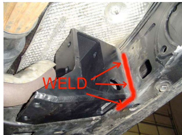
D.S. Bracket Welded in Place
