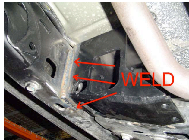
P.S. Bracket Welded in Place
