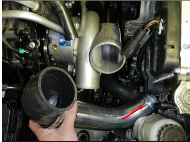
2) Thread piping through previously cut holes
