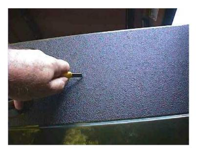
NOTE: The "Clear Frost" colored Protectors will take a week or so (faster in warm temperatures) before the clear color will even out, the adhesive is very thick and viscous and it takes time for the adhesive to fully "wet out". Please do not be alarmed if, directly after application, the Protector looks spotty, you are only seeing the adhesive through the clear material.
