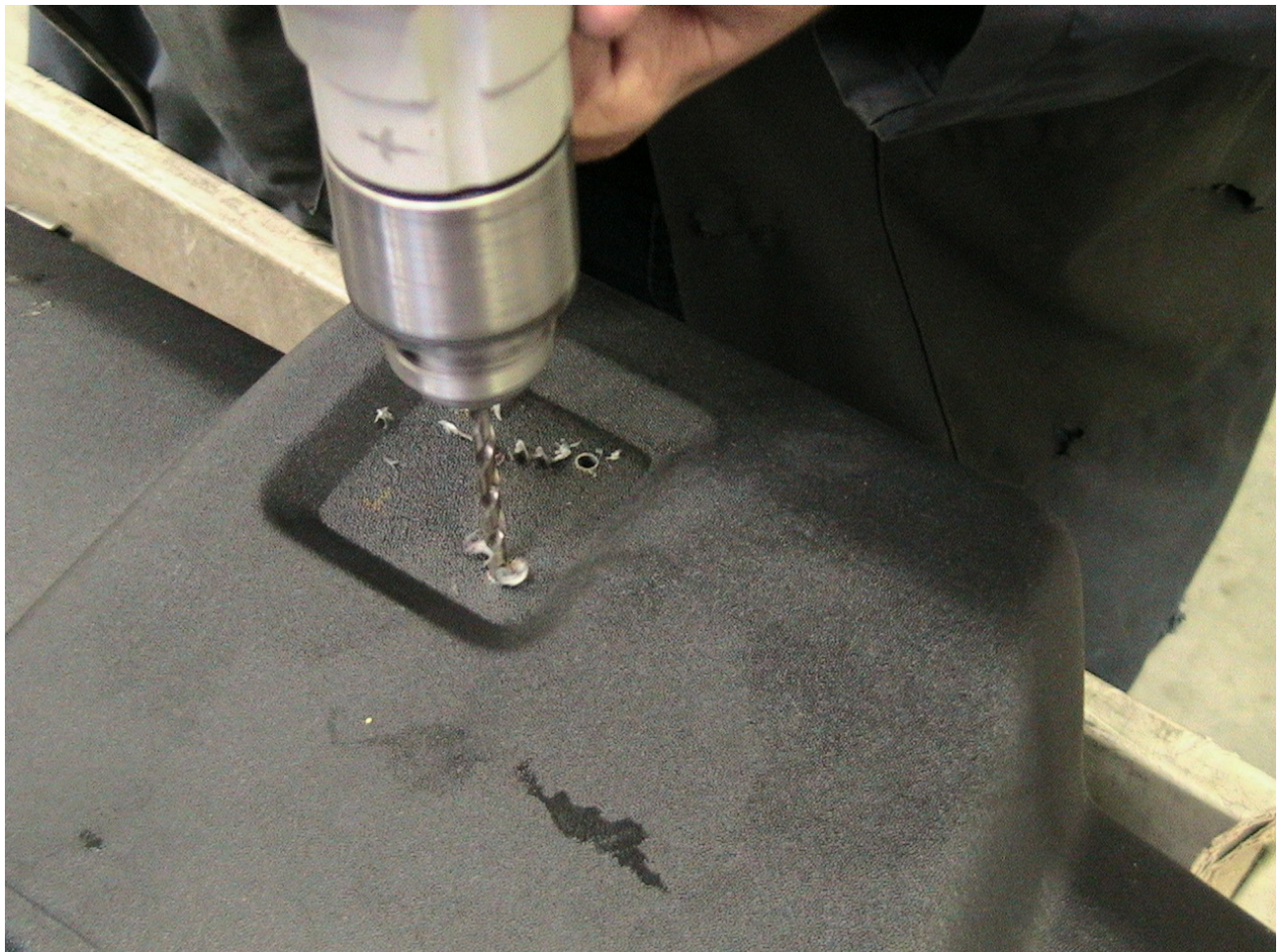
Figure 3: Drill corners of tow hook cutout
