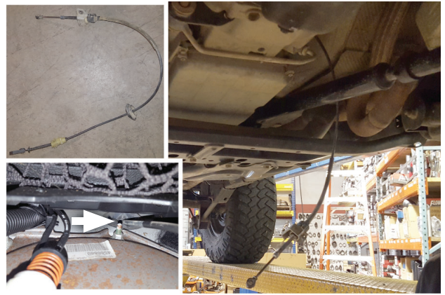
15. Working in cab and under vehicle, thread shifter cable through hole into transmission tunnel and remove it from vehicle.
