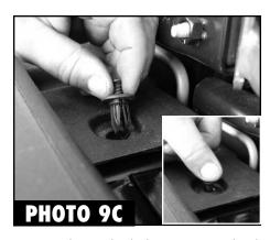
**9C** Insert the two clips back into position and push them down into place. (See Photo 9C)
