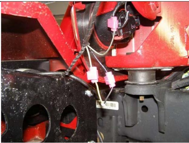
29. a) Feed loom down until LHS indicator spliced wiring is in position to be attached to vehicle indicator.
