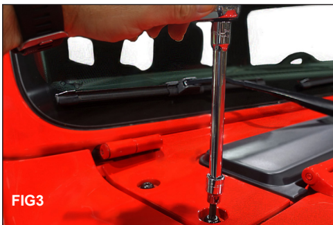
(FIG3) Using a T40 Torx bit socket remove the 4 Cowl mounting screws and carefully remove the Cowl. (FIG4) Run the wiring for the cube lights then re-install the Cowl. Using a T40 Torx bit socket loosely install 3 of the Cowl mounting screws.
