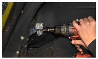
**22.** Install a 1/4-20 nut-sert into the hole that was just drilled out in the previous step. Again, we recommend the use of a professional nut-sert installation tool.
