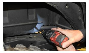
7. The next existing hole to be drilled out is located at the opposite end of the wheel well, above where the frame rail bends downward, as shown below. Drill this hole out to 25/64"
