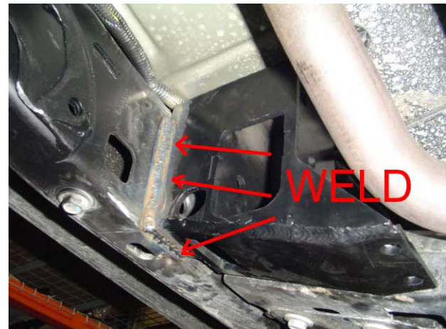
P.S. Bracket Welded in Place
