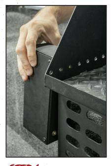
Line up the holes to the ammo can tray with the rivet nuts in the back pane of the Power Panel.
