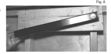
install cross braces using provided screws (HAT-050). Install the two pulleys (HAT-116) using screws (HAT-125) on cross braces 32 inches apart (Fig. G-I) with 1/2" offset. Keep in mind that the center of the pulleys is your lifting point for removing the top.
