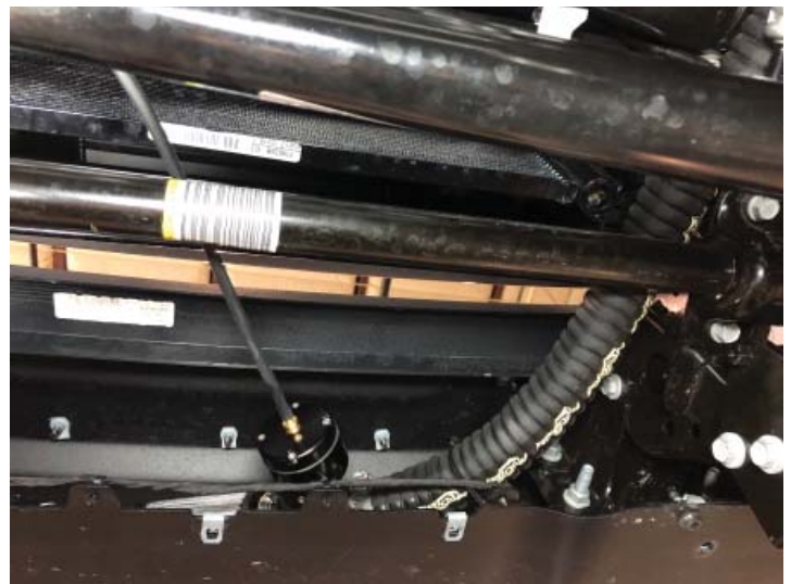
Surge Valve Installed
