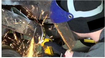
Once you've cut the body mount bracket free, remove the body mount bushing as it will be used during the replacement install.
