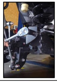
**4.** Using an 18mm socket and wrench, remove lower bolts to sway bar links. **Do not discard factory hardware.** Repeat for other side.
