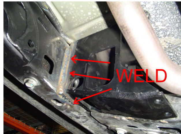
P.S. Bracket Welded in Place
