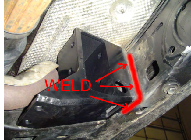
D.S. Bracket Welded in Place
