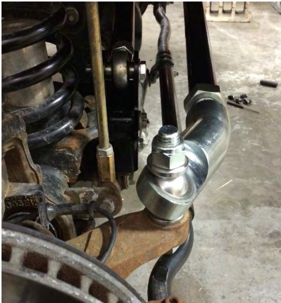
Passenger side knuckle connection
