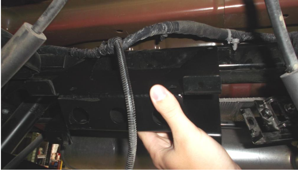
Figure 5. Installing Air Tank Mount
